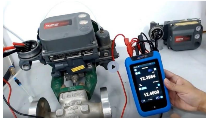
Figure 2: Additel 227 Communicating via HART with a Field Vue valve positioner.
